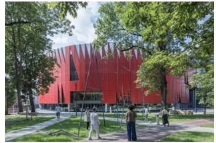
(3) CH+K_Jihlava Municipal Arena_credit Laurian Ghinitoiu 3.jpg
